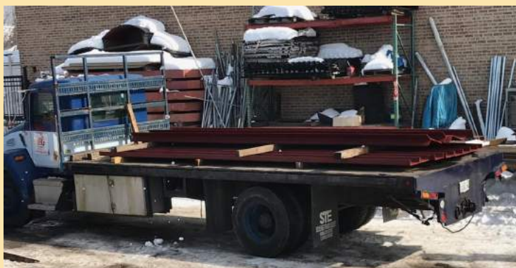
Left: Delivery of the final pieces of steel.
